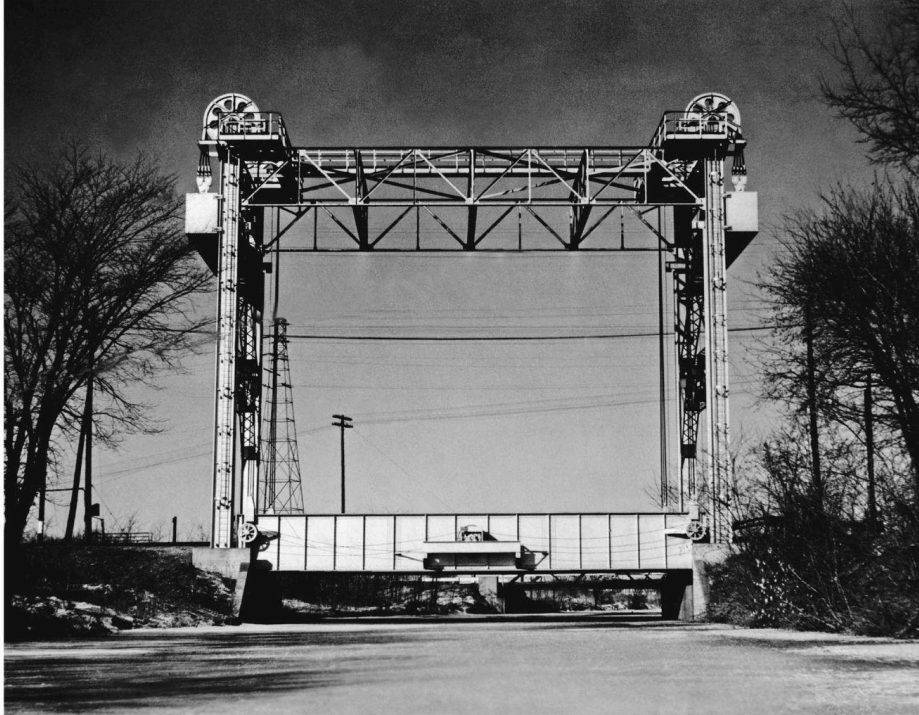
The entire bridge and tracks were lifted vertically 30 feet into the air, so boats could go under.
