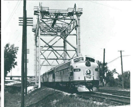
The Morning Hiawatha rumbles over the Portage Canal bridge. In this June 1961 scene, the two 85-ton counterweights have been removed from the bridge superstructure, which itself will be dismantled seven years later.
